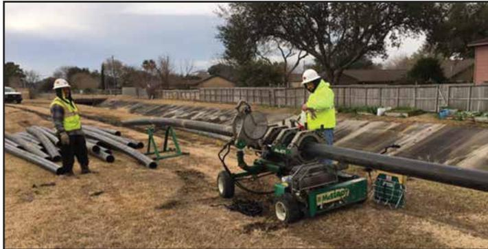
Pipe bursting is a method of replacing buried pipelines – such as water lines - without the need for a traditional construction trench. The process involves pulling a new pipe through an existing pipe using expansion tools powered by hydraulic generators. According to Assistant Public Works Director Brent Costlow, projects completed using pipe bursting reduce the overall cost by 35-40% on average.
